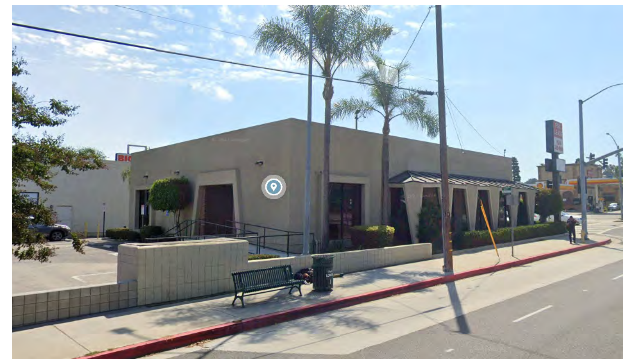
NORTHWEST CORNER LOOKING TOWARDS THE BUILDING ENTRY
