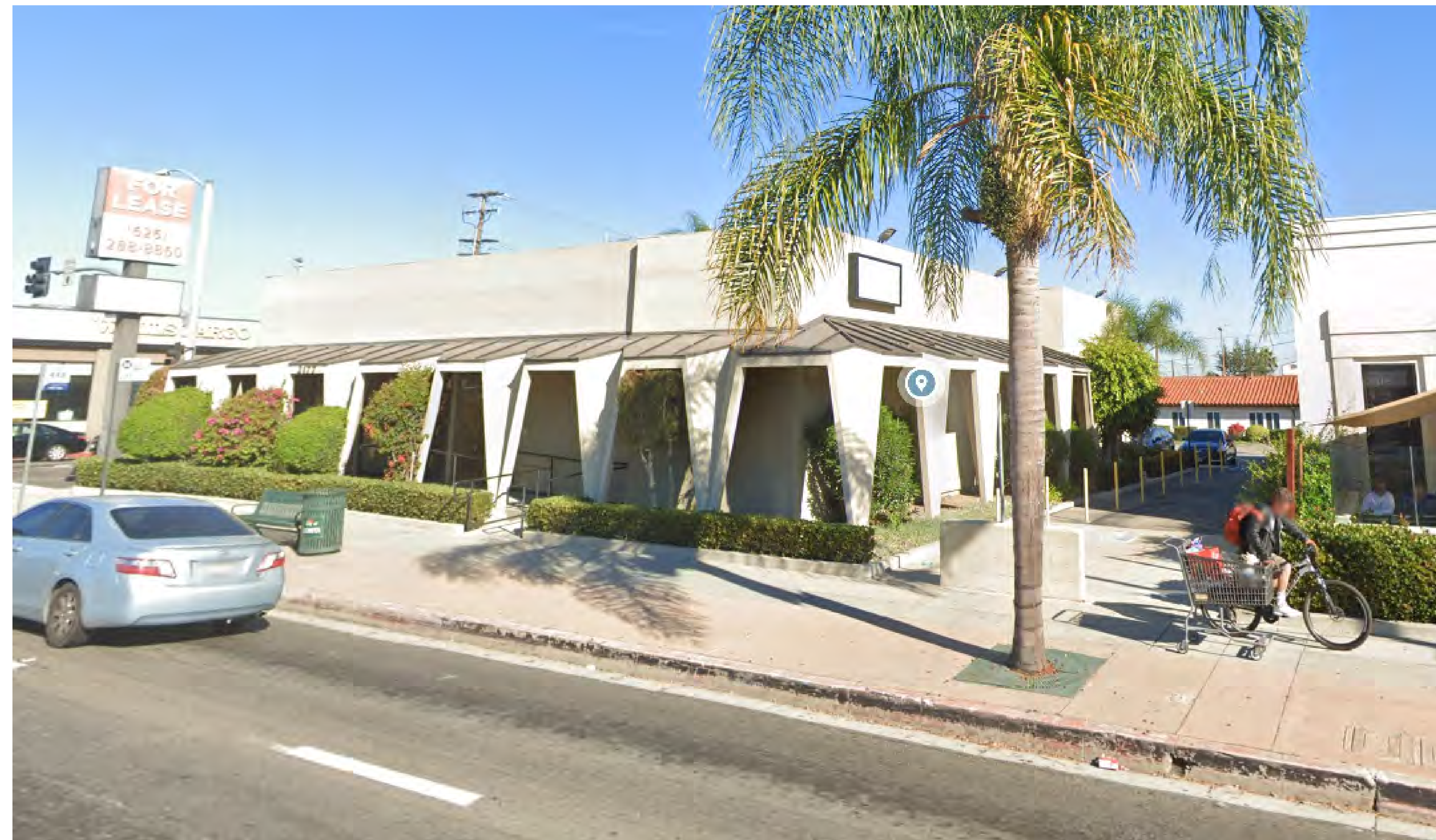
SOUTHEAST CORNER LOOKING TOWARDS THE BACK OF THE BUILDING
