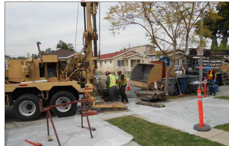
Typical Hollow Stem Auger Set-Up for Deeper Borings
