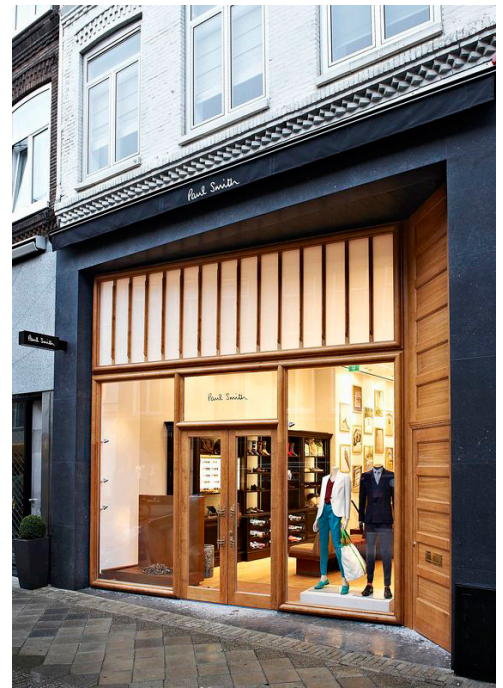
New storefront within a traditional context
