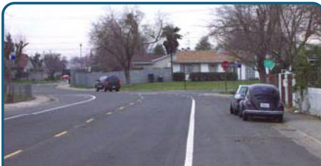
Example of edge line striping for on street parking
