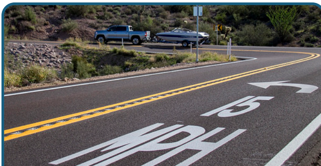
Example of speed legends in a turning lane
