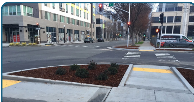
Example of a curb extension (bulbout) at a crossing
