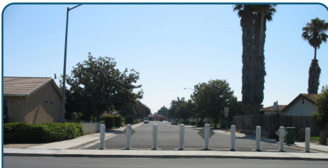
Example of a full closure for access control
