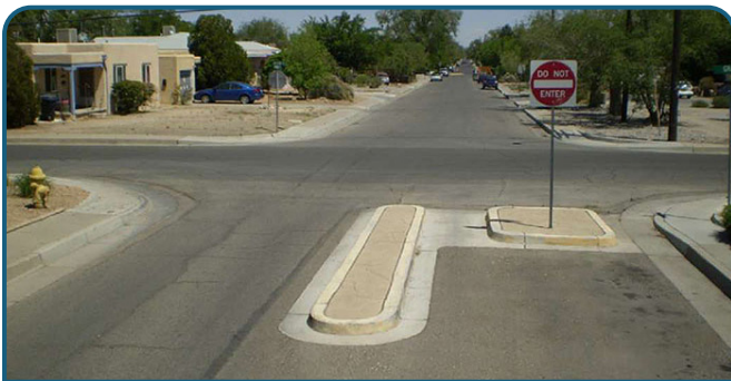
Example of a partial closure
