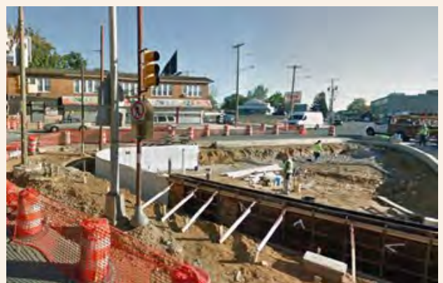
Hazen coordinating with contractors during ROW GI construction in Philadelphia.
