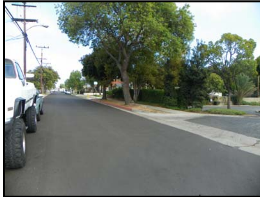
Citywide Slurry Seal Project – 242 nd Street
